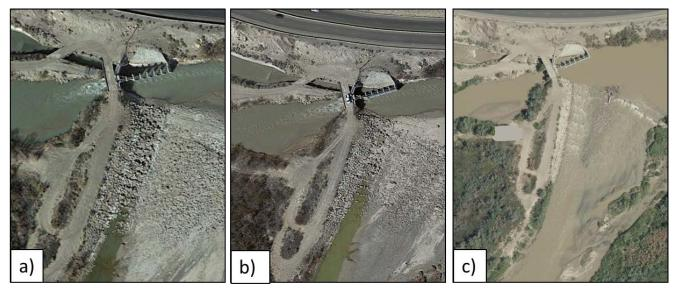
Figure 17. Hogback diversion and fish passage (natural-like boulders). Dry when sluicegates opened and river flow at or below 1,000 cfs; a) 700 cfs, November 2013, b) 1000 cfs, March 2015, c) 730 cfs, August 2016 (sluicegates appear closed).
