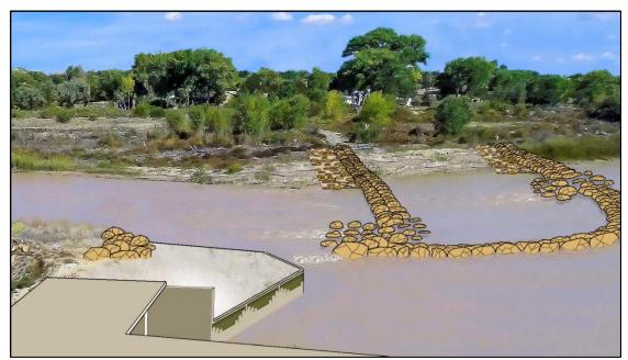
Figure 6. Conceptual design of Fruitland-Cambridge grouted diversion dam with fish passage integrated into each of the two-step boulder fields (NNDWR 2016).
